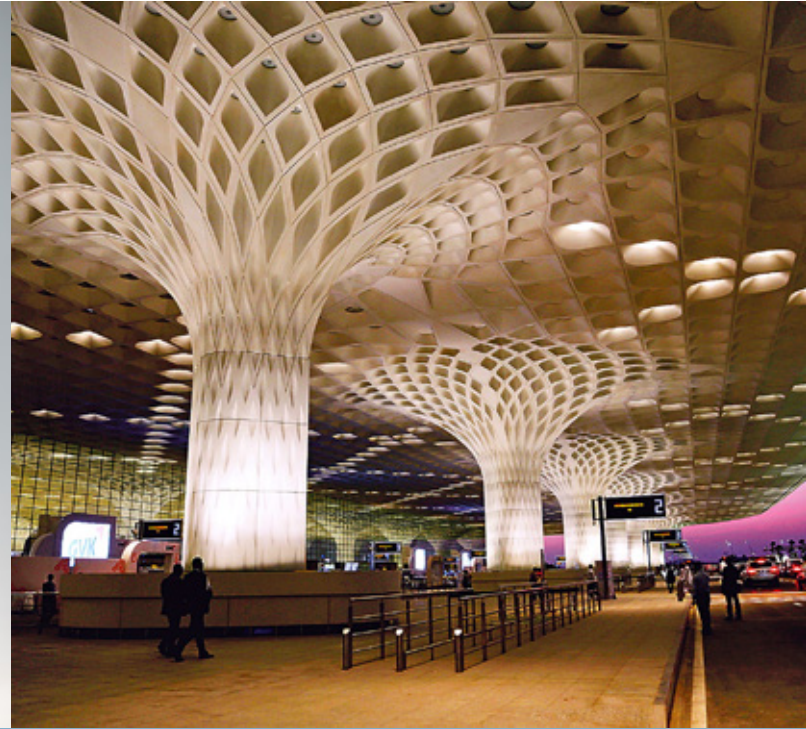
A terminal building of Chhatrapati Shivaji Maharaj International Airport in Mumbai, India, where ARG Fiber was used in the ceilings and pillars Photo: Courtesy of Nippon Electric Glass Co.,Ltd.
