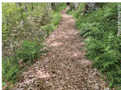
A walking road paved with Japanese cypress wood chips
