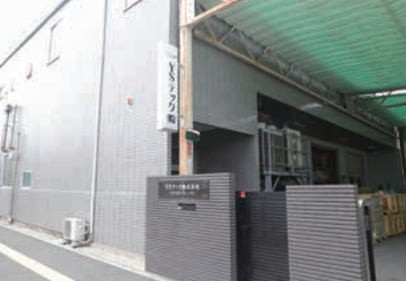
YStech Co., Ltd. - Head Office (Suita City, Osaka Prefecture)
