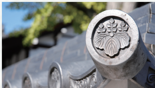
Kamon crests can also be seen adorning yane-gawara roof tiles used in Japanese structures, including castles, temples, shrines, and houses built with traditional techniques. Shown in the photo is a kiri-mon 4 crest.
