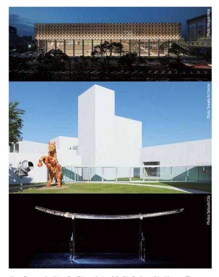
Above: Renowned architect Ban Shigeru designed the Oita Prefectural Art Museum. The building's beautiful latticed appearance was created using the bamboo art *henso*, a technique for weaving bamboo strips into a precise pattern.
